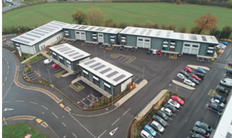
Phase 1 - NiPark, Newport
